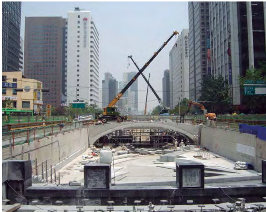
Figure 13.13: The upper panel shows restoration work in progress on the Cheong Gye Cheon in Seoul (on June 24, 2005). Two years later (lower panel on June 7, 2007), water is flowing where a freeway once passed over the top of the river's course. Vegetation blankets sections of the restored bank and people stroll or sit along the edge of the waterway, once a contaminated drain
