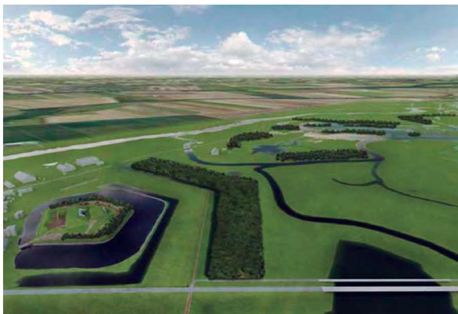
Figure 13.12: The Noordwaard polder project includes “through-flow” areas and green wave-inhibiting dikes that are up to 65 cm lower than the original engineered dikes. Through-flow areas serve to divert some of the higher flows and reduce discharge volumes during winter. This involves a shift in concept from constraining all water in the channel using high levee banks to lowering the levees and allowing floodwater to spread out onto the floodplain but using levee banks to protect houses and infrastructure
